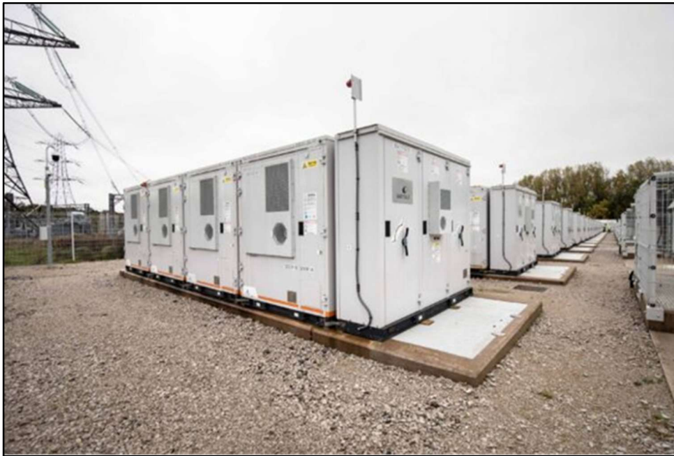
Plate 3.10: Example of the construction of BESS Compound
